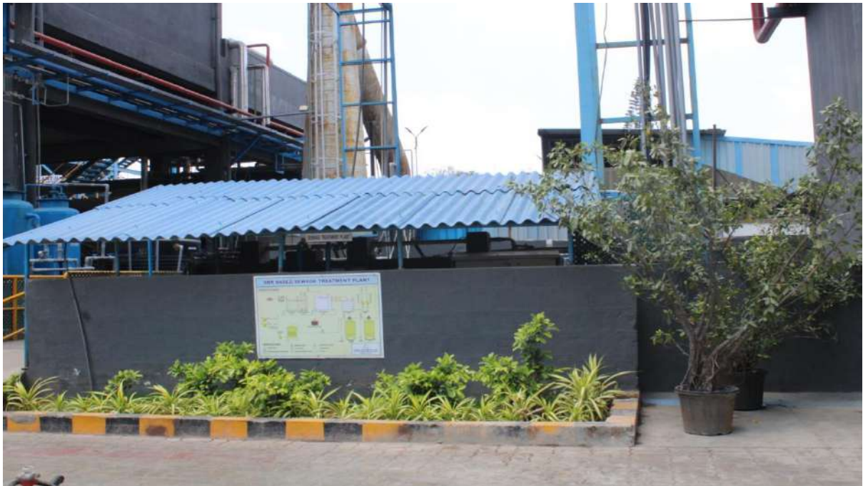
View Of STP
